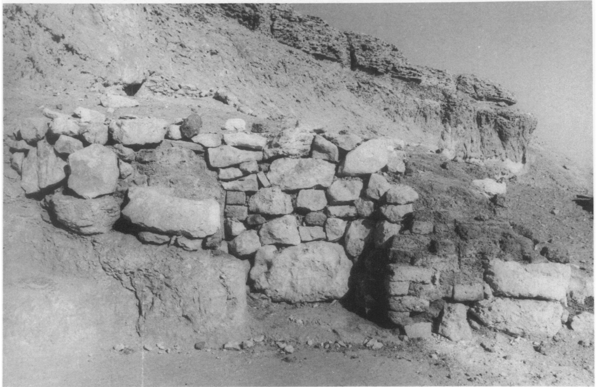
2. Tell el-Amarna: detail of an entrance in a wall built of mudbrick, fired red brick and stone against the south side of the forecourt of tomb 6, looking south. The blocking is modern
